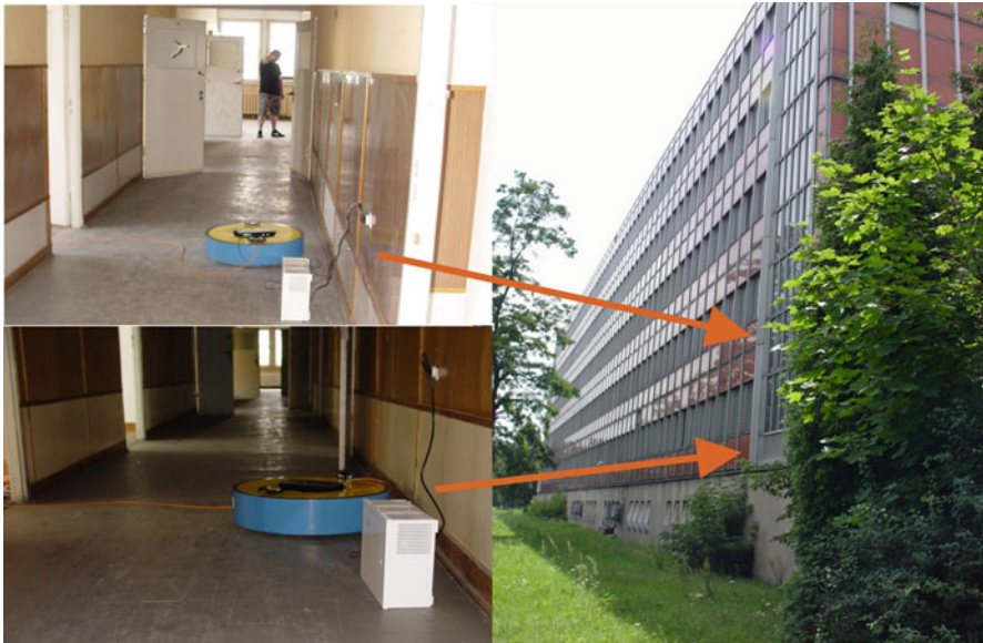
Fig. 23.6 The general view of the building used for monitoring of its rotation moving via AFORS-2. Left picture shows AFORS-2 mounted in 2nd and 1st building layers
